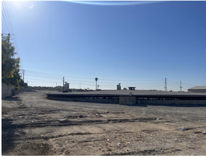
Photograph 1: View looking southeast along western boundary of Project site.
